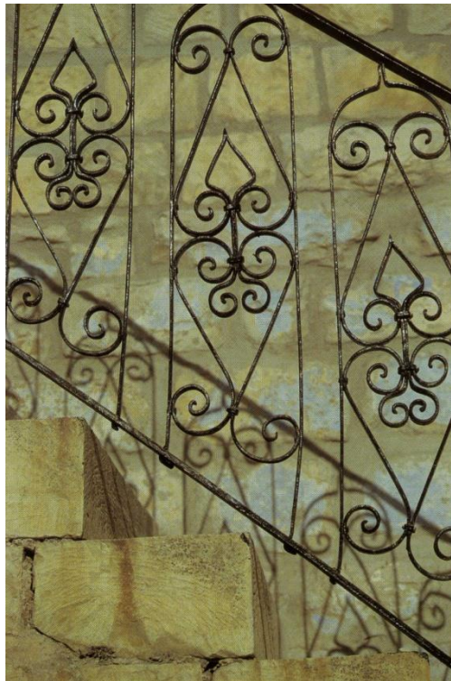
Photo 7. Iron protection on stairs in Shamma house in Safad 13
