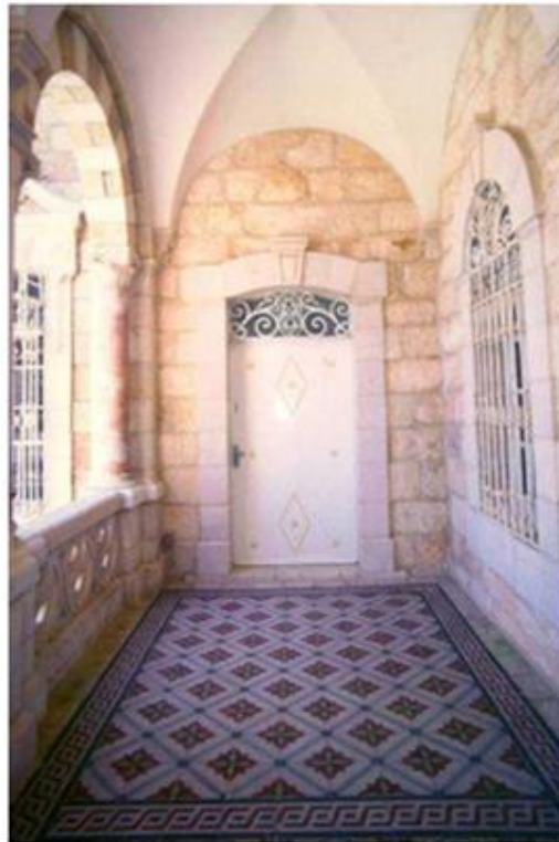
Photo 12. Application of the traditional floor tiles in the entrance hall 28
