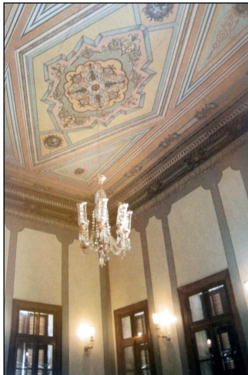
Photo 9. Some woodwork in the roof Agha Tuqan house in Nablus 24
