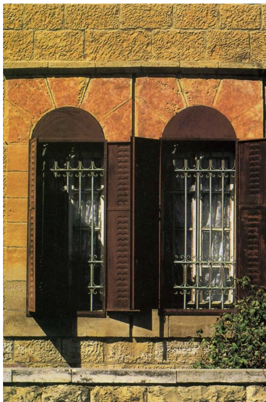
Photo 1. Formations arches on the windows in Yakoub El-Zarour house in Ramallah 7
