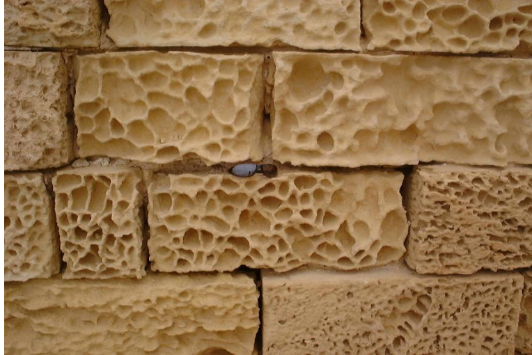
Figure 1. Salt weathering of building stone on the island of Gozo, Malta https://commons.wikimedia.org/wiki/File:Salt_weathering_in_gozo.jpg
