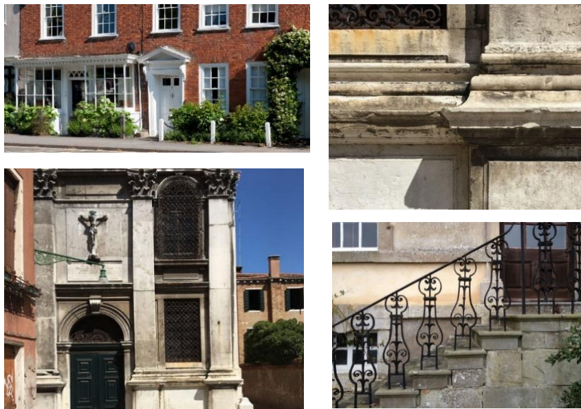
Figure 11. Top left, Brick house in Dedham, Essex, UK. Top right, Stone base and pedestal in Venice. Bottom left, Church façade in Venice. Exterior stairs at Frampton Court, Gloucestershire, UK Images courtesy Francis Terry
