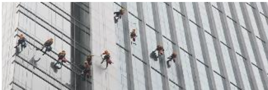
Figure 5. Window cleaners working on a glass high-rise building https://www.istockphoto.com/video/skyscraper-cleaning-gm472794299-15167907
