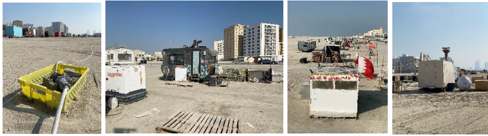
Figure 3. Examples of the problems due to improper infrastructure networks
