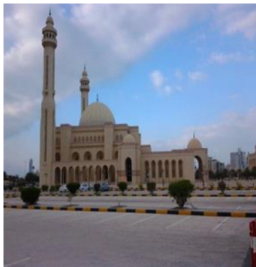
Image of the overall volume of the mosque
