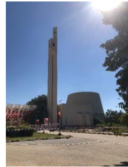
Figure 3. A minaret, a landmark to identify the mosque location (the researcher)
