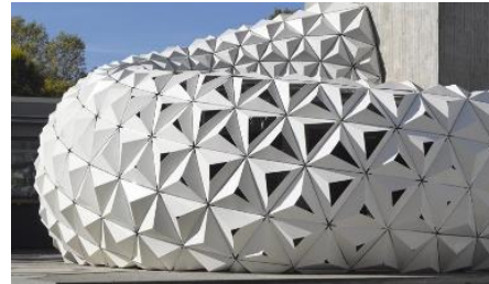
Figure 6. Biopolymer facade system (Köhler-Hammer & Knippers, 2014)
