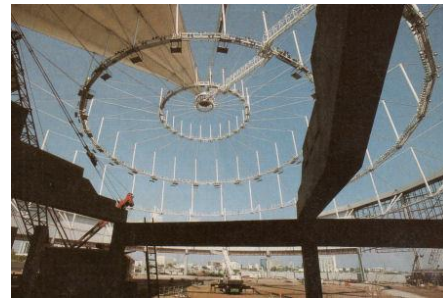
Figure 13. Florida Suncoast Dome (Saint Petersburg, USA), 1989 (photo: Case Western Reserve University)
