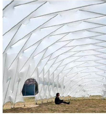
Figure 11. Moom: a tensegrity-based experimental tent 2011, Tokyo University of Science (photo: The Japan Architect, 84)
