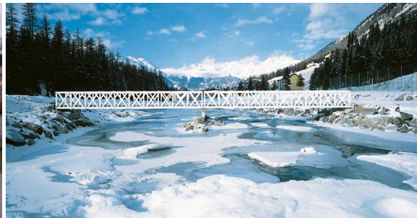
Figure 4. GFRP bridge in Pontresina Bridge, Switzerland (Smits, 2016)
